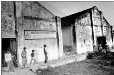
The first home of CRP – cement store houses in the grounds of Dhaka Hospital
